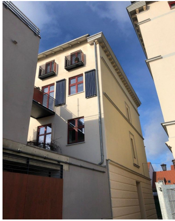
Fig. 2.2. Solar panels on the wall of the house (Stralsund).
