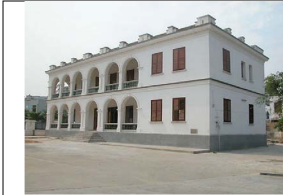
Figure 57: Former British consulate building in Beihai, south China 289 .
