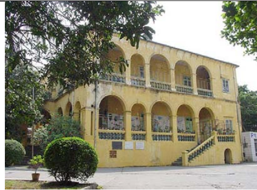
Figure 58: Former German consulate building in Beihai, south China 290 .
