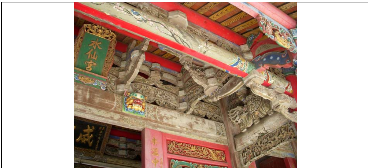
Figure 70: The color of timber painting in entrance hall. (Author)
