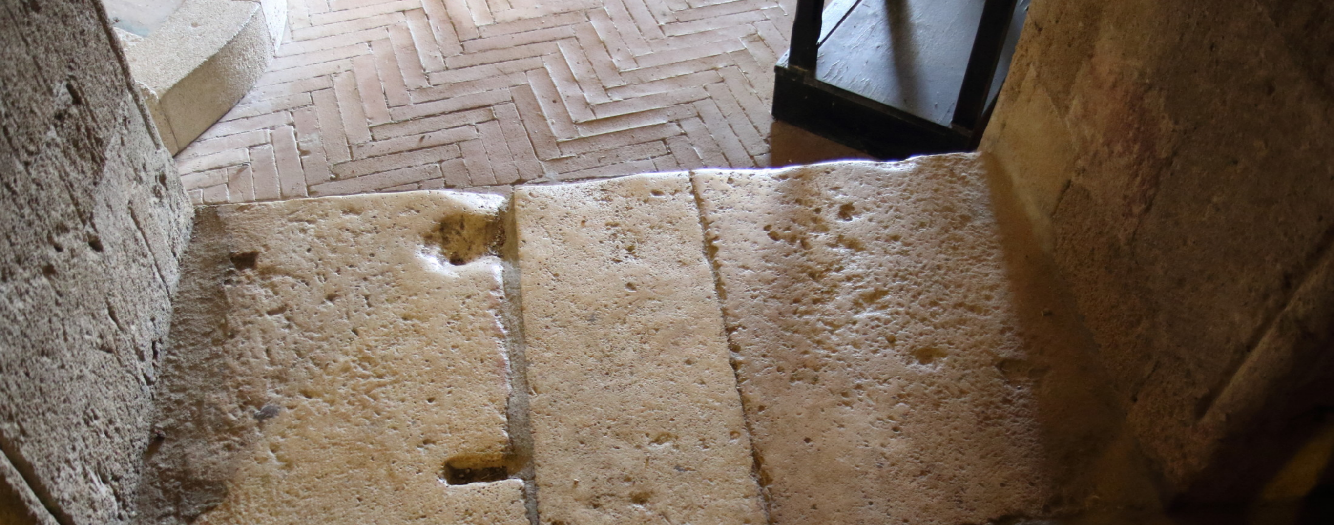
Rounded edges in re-used antique slabs serving as door-steps
