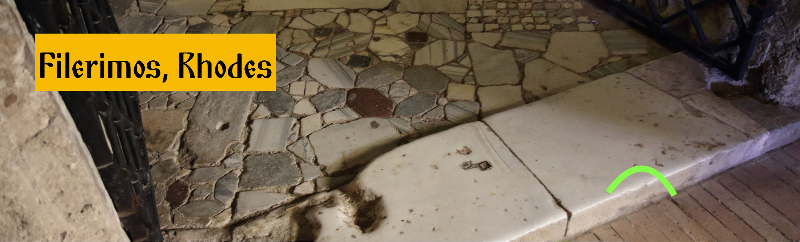
Rounded edges in re-used antique slabs serving as door-steps
