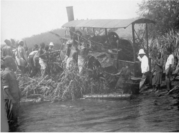
Figure 5: Steam Plough Sunk in Mukondoa River.
