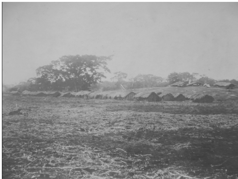
Figure 7: First workers' camp in Kilossa.
