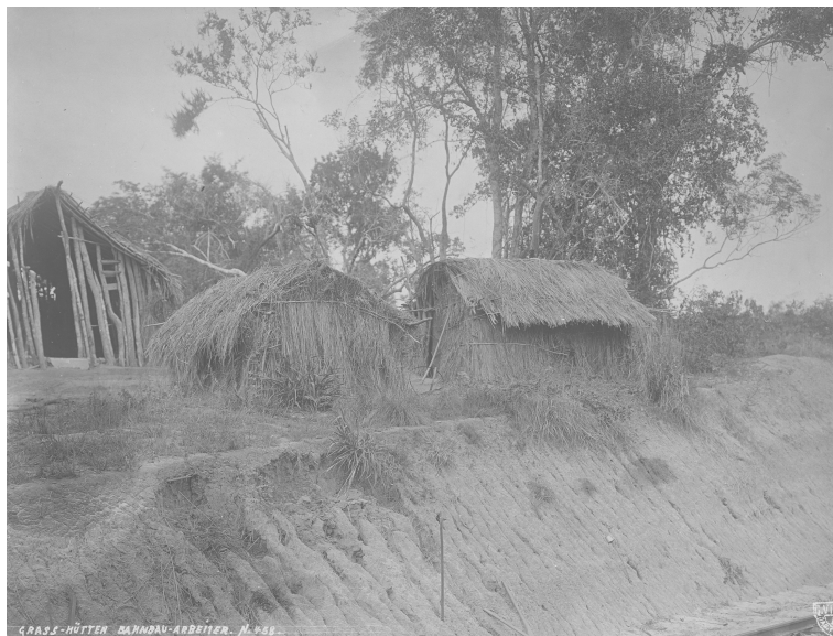
Figure 4: English: “Grass huts of railway workers, no. 458”.
