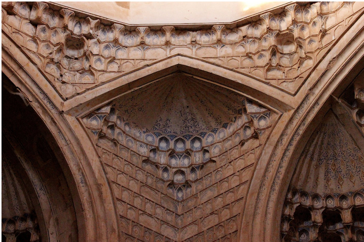
Figure 21. Recently restored wall painting repertoire in the entrance chambers of the Madrasa Ghiyasiyya of Kharghird (1441–1442) (Ana Marija Grbanovic).
