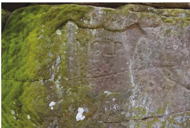
Figure 6. Almost illegible graffiti due to biological coating.
