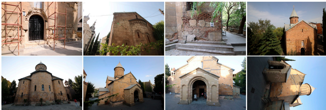
Figure 5. Example images of terrestrial photogrammetry: top row Lurdji; bottom row Sioni.
