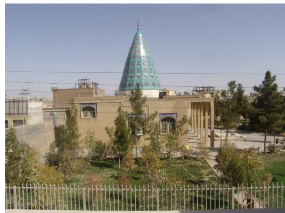
Image 4- Southern facade and the mausoleum's surroundings (Source: Archive of ICHTO)
