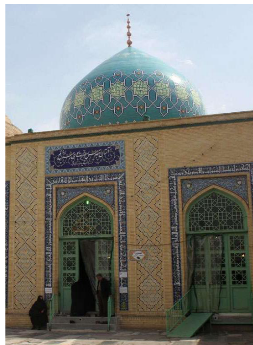
Image 4- Entrance and new dome of the mausoleum of Mūsā Mobarqa'
