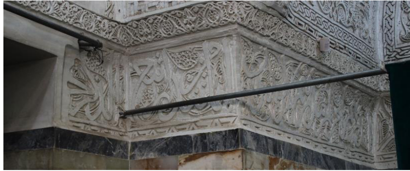
Image 22- The inscription band on the northern side and the demolished part on the present entrance
