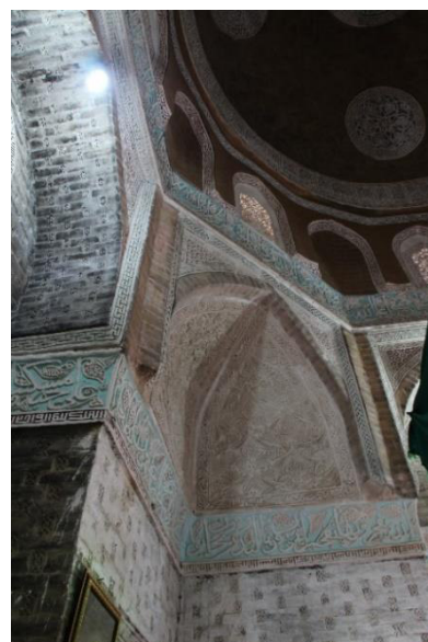
Image 16- Interior of domed chamber, looking SE
