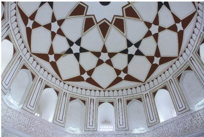
Image 16. Rectangular panels with pointed arch on collar of the dome zone (source: Archive of OOQ)
