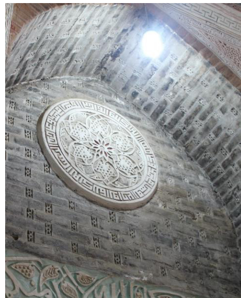
Image 45- false bricks on W chamber
