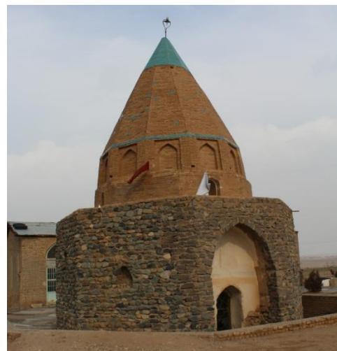
Image 8- Southern side of the tower
