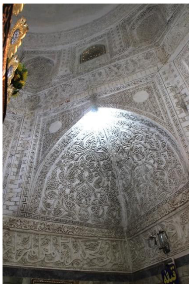
Image 17- view of squinch area in dome chamber
