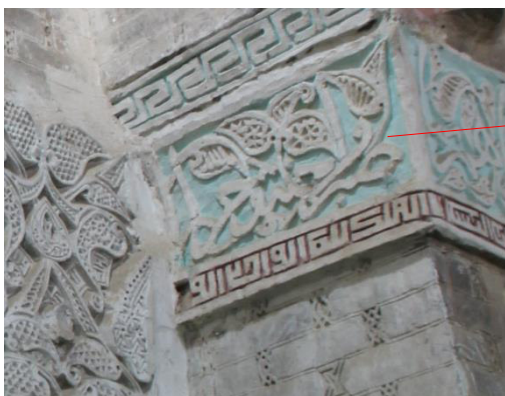
Image 21-22. Southern side and details of the inscription as it connects to the additional wall on the mihṛāb side
