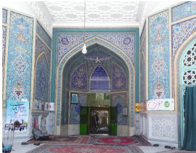
Image 9- Current appearance of the entrance porch
