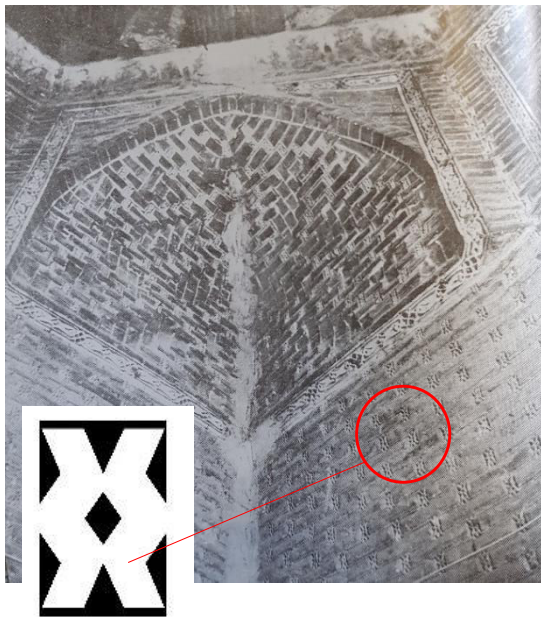
Image 13- Joint plugs on walls (Source: TP , fig.7)
