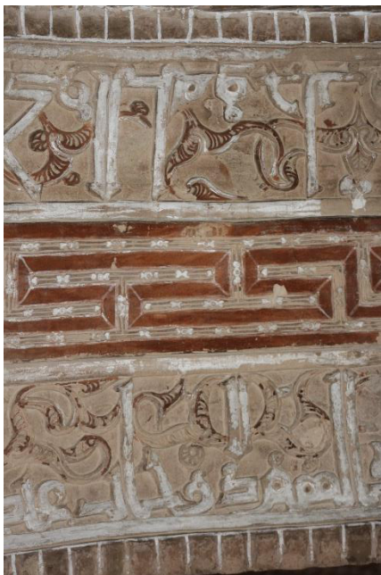
Image 31. Detail of colored plaster work on soffit of Ardestān mosque (source: I. Āqāğānī, 2015)
