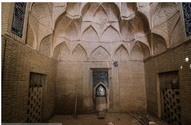
Image 10. Interior of the mausoleum of Bābā Qāsem at Eṣfahān ,1340 (source: esfahanemrooz site, date: 25.08.2019)
