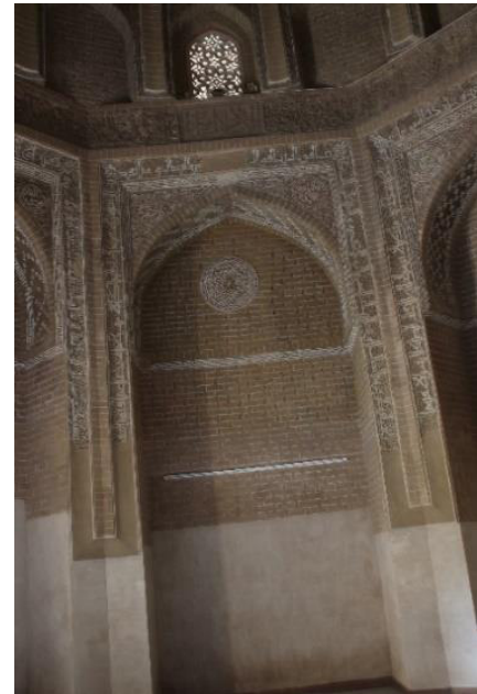
Image 11. The present condition of the east doorway
