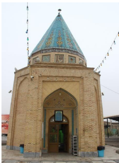
Image 5-The portal after restoration, 2017 (Source: Archive of OOOQ.)
