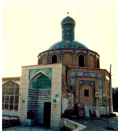
Image 12- Entrance facade of the N doorway, 1990 (source: Archive of OOQ.)
