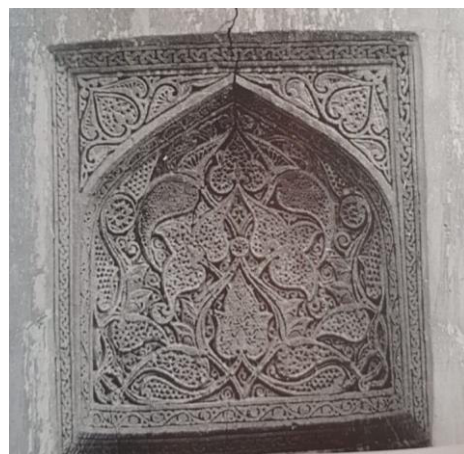
Image 7- One of the niches on the northern wall of the hallway (Source: Raḥmatī, p.92, with additions by the author)
