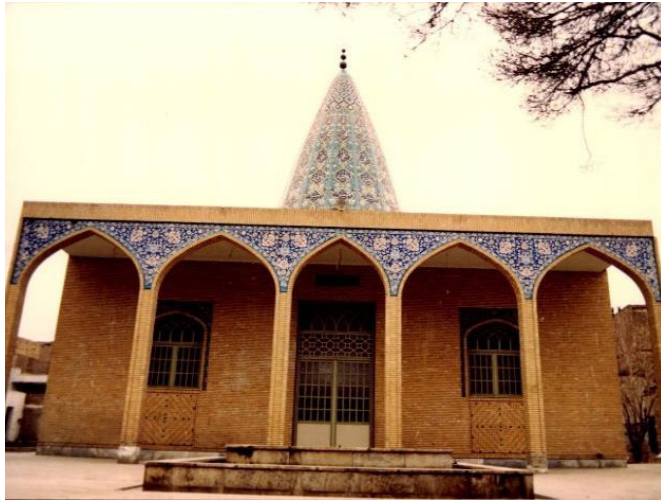
Image 5- Eastern façade (Source: Archive of ICHTO)
