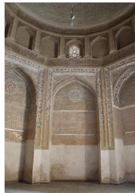
Image 13. The present condition of the west doorway
