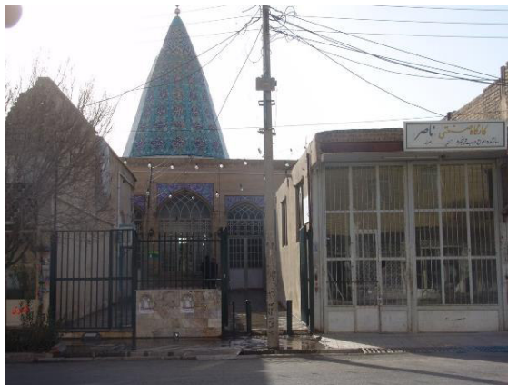
Image 3- Western facade, the entrance of the complex from the street (Source: Archive of ICHTO)
