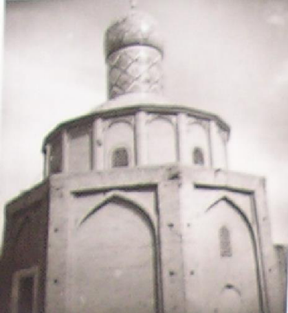
Image 7- Exterior of the mausoleum in 1970, (Source: Archive of ICHTO)
