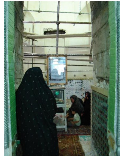
Image 6- Domed chamber in the course of restoration 2001 (Source: Archive of ICHTO)
