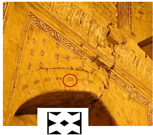
Image 32- Horizontal brick-end plugs, before restoration (Source: Archive of ICHTO)
