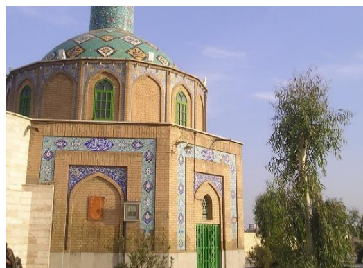
Image 6- External facade of the building
