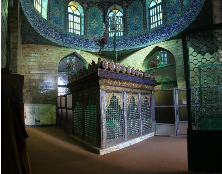
Image 24- The Existing condition of the domed square and new shrine
