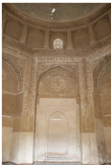
Image 19. the present condition of the south side and the mihrab
