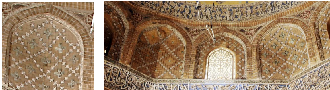
Image 26. simulated incised brick joints on the inner frames of blind niches in lower part
