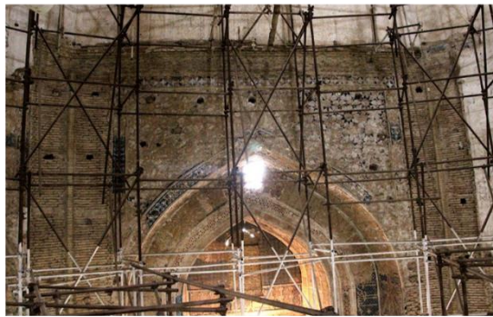
Scaffolding remains and the first decorative phase.
