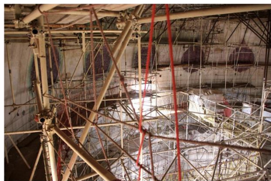
Scaffolding remains penetrating first and second decorative layer. The modern scaffolding in the interior of the mausoleum.
