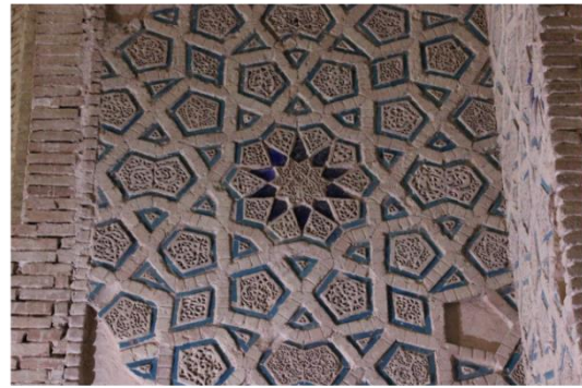
The first decorative stage: ceramic revetments.
