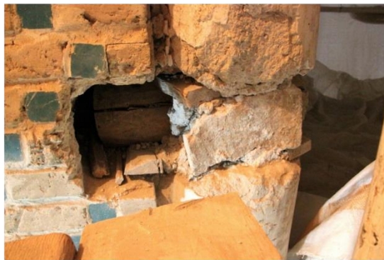
Scaffolding remains penetrating first and second decorative layer. The modern scaffolding in the interior of the mausoleum.
