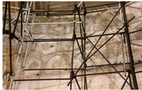
Scaffolding remains and the second decorative phase.
