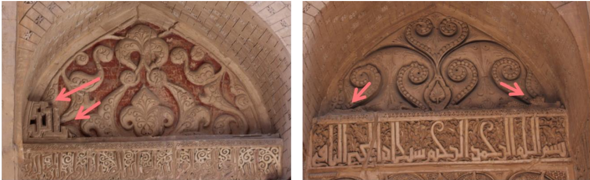
The Pir-i Bakran mausoleum: perforated stucco grills (only fragments remain) from the third decorative phase 1312-3, were made to cover earlier stucco revetments from the second decorative phase (1302-3).
