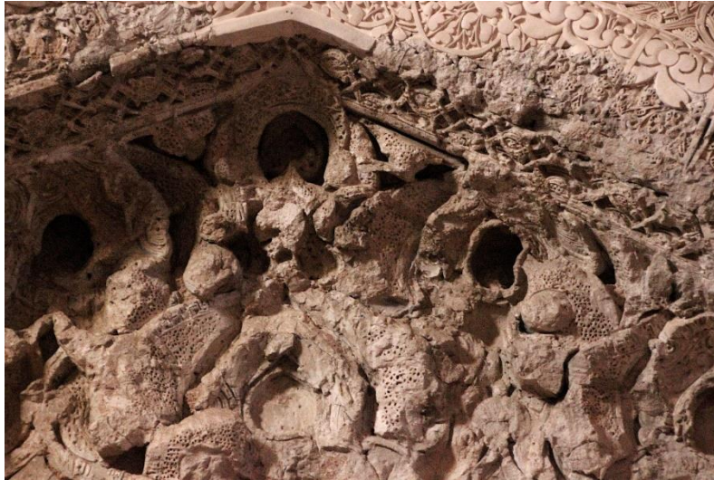
Figure 28: Detail of the monumental lunette of the Tabriz Friday mosque mihrab: it is formed by an accumulation of constructed hollow elements.
