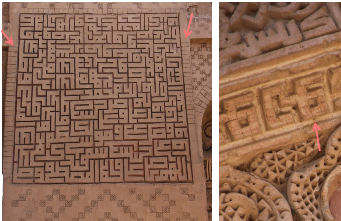
Figure 71: Examples of use of gridlines for Square Kufic inscription design transfer into carved stucco medium (left: the Pir-i Bakran mausoleum; right: the Haftshuya Friday mosque mihrab).
