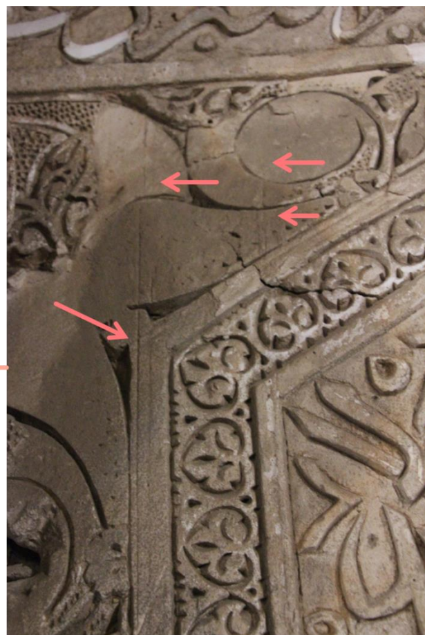
Figure 18: Example of architectural lines, direct incisions with ruler, on the unrestored parts of the carved stucco mihrab of the Marand Friday mosque (Cat. No. 22).
