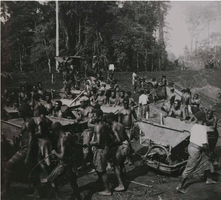
Figure 1. ‘Construction of the Central Railway 1912–1914. Apparently moving the tipper waggons to a new Shaft. [...]’.
