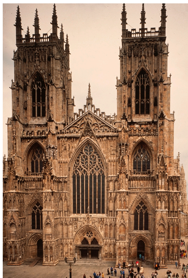
Ill. 4 The west façade of York Minster c. 1990
