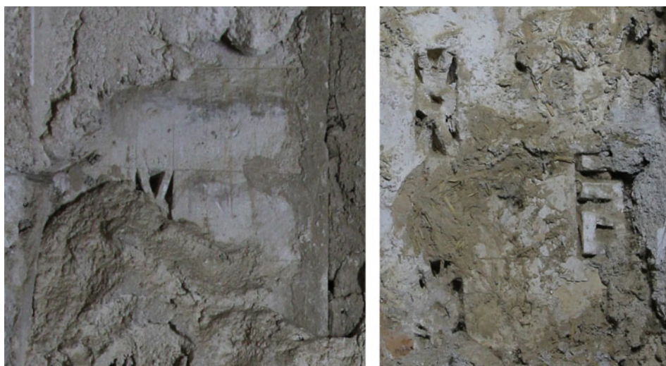
Fig. 8. Incised construction lines in the earliest phase of brick decoration to the right of the mihrab niche (L), and square Kufic Allah brick plug (R).
