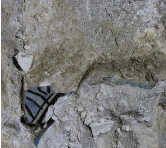
Fig. 10. Fragment of eight-pointed glazed half star tile from the dado wall revetment of the shrine.
