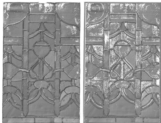
Figure 4. Juxtaposition of window nX4b from Koszewko before (left) and after the conservation (right).
