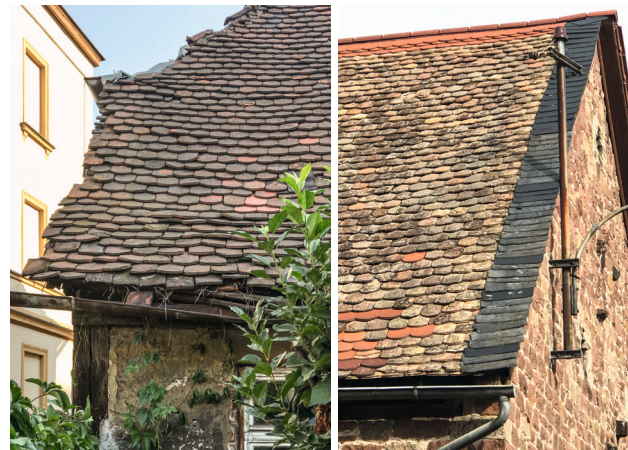
Fig. 5: Total loss (left); preservation, repair and careful addition (right) [Schalk 2018].
