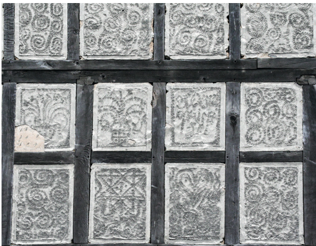
Fig. 2: Großropperhausen, municipality of Frielendorf, Hesse; barn wall with rich ornamentation in the panel sections [Scherb 2006].
