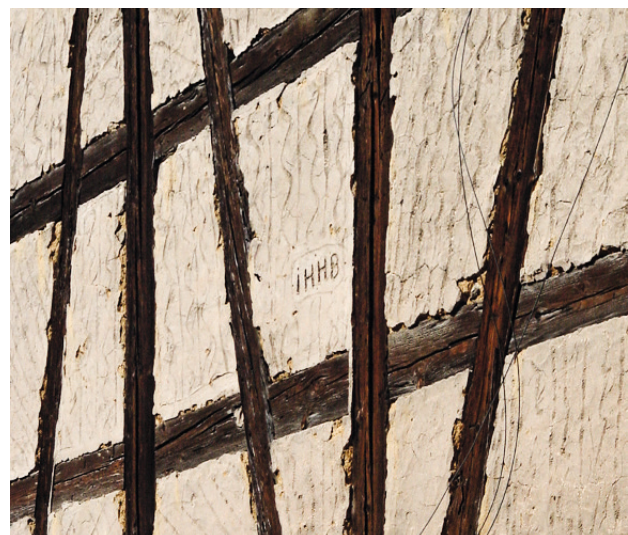
Fig. 4: Bonigen, Filderstadt, Württemberg, Haupt Strasse 7A, gable barn with wavy bands 2nd half of the 18th century [Marstaller 2017].
