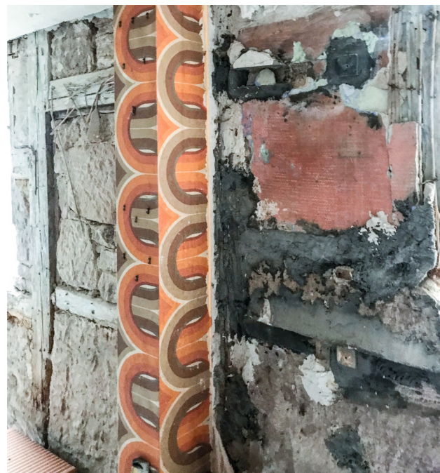
Fig. 7: Demolition or preservation of living environments? [Schalk 2018]
