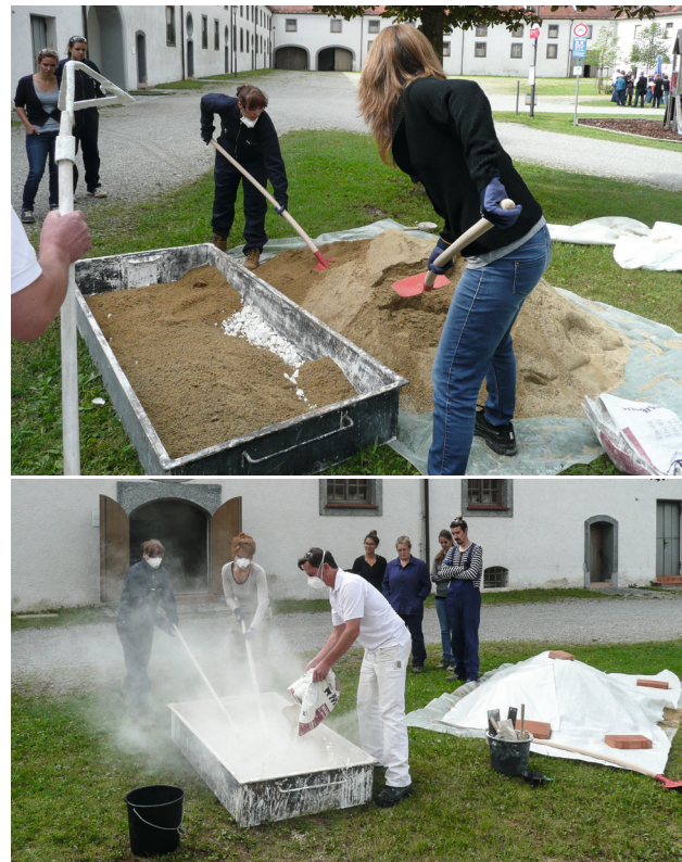
Fig. 3: Intensive week Building Archive Thierhaupten; production of dry-erased lime mortar in the mortar trough by adding layered lime and sand (top); extinguishing the lime; the resultant heat leads to water vapour formation (below) [Wenderoth 2018].
