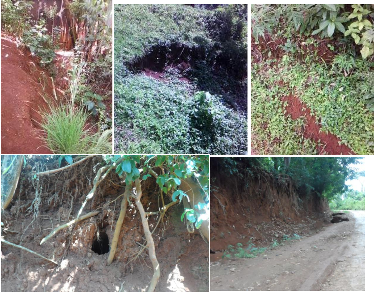
Figure 6.11: Cracks observed before landslide occurrence.
