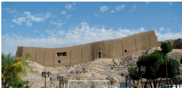
Image 4-115: Restored Rampart of Rayy in Češme 'Ali, View of Southeast (Source: Author-2011)
