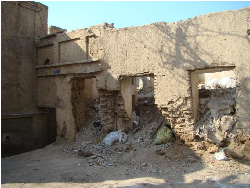
Image 5-25: Widespread Destruction in Historical Areas (Source: Author-2012)
