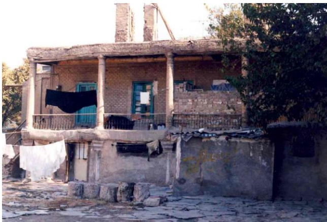
Image 4-141: The remains of the eastern building in the Malek garden (Source: Afrund: Gozāreš-e Pažuheši va Barresi va Šenāsā'i-e Āsār-e Bāstāni va Tārihi )
