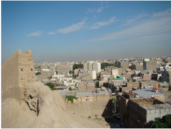
Image 5-8: Constructing a Building next to the Ancient Wall of the City (Source: Author-2012)
