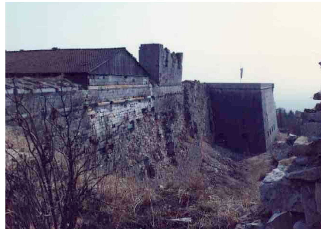
F 200 Bastion Schnaittach
