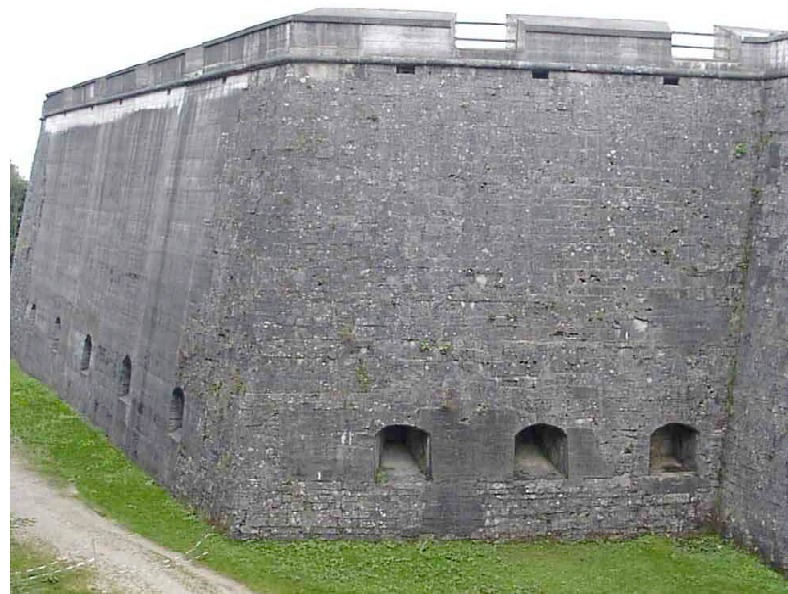
R 20 Bastion Karl F 452 2002 S.Thole
