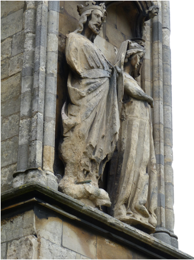
Ill. 16 Lincoln, Cathedral, Angel Choir, buttress figures, “Edward and Eleanor”, note the lack of support under their feet
