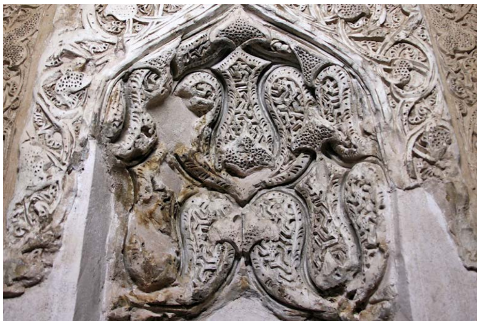
Fig. 4: An example of pseudo-undercut stucco relief from the Miyandih mosque in Qamsar (interior lunette of the mihrab)
