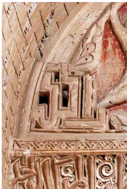
Fig. 7: Detail showing the remains of the perforated stucco grill at the Pir-i Bakran mausoleum (3 rd decorative stage; 1312-13 CE)
