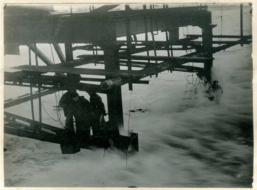
Figure 2. Carpenters attach the pipe tension ('Rohrspannung') in heavy seas, July 1912.
