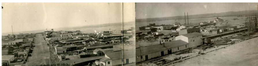
Figure 1. Storage and accommodation of the construction site with Swakopmund in the background.
