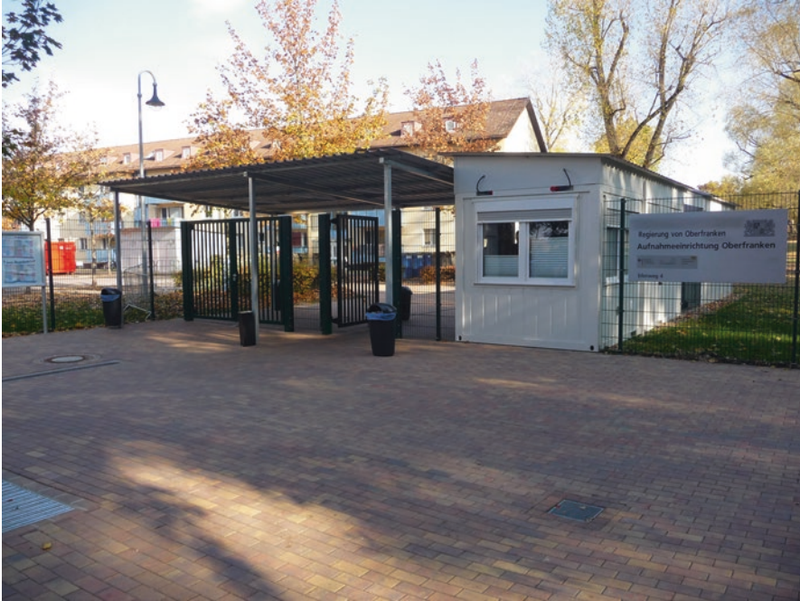
Fig. 4.2 Checkpoint and entrance control at Bamberg's AEO; in the background one of the residential buildings. (Photo by author, 21 Oct. 2018)
