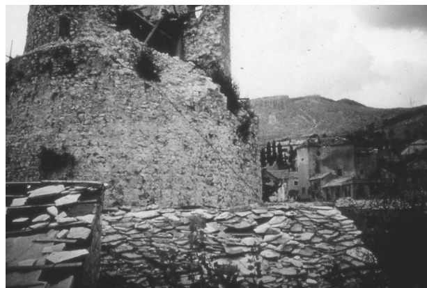
2 The destroyed tower at the foot of the Mostar Old Bridge
