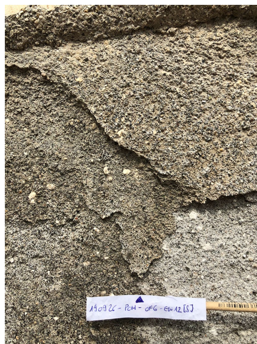
Fig. 13 Tomb EN12, south facade. Detail of the sampling area of the crust formed at the surface of the arriccio render layer
