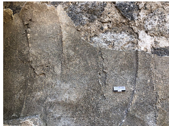
Fig. 7 Tomb PN-EN12, east facade. Detail of the surface of render layer arriccio 0. Traces of the working tools left after the application of the mortar are clearly visible
